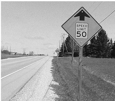
REDUCED SPEED AHEAD SIGNS also may be used to give advance warning of a lower speed zone. This sign should be used in rural areas to alert motorists when they need extra time to slow to the posted limit.
