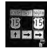
inspection findings on a list of signs. The inspection team should drive the road in both directions to view signs as the driving public
