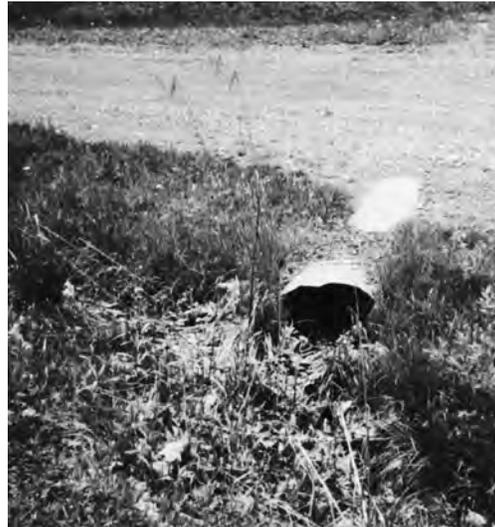
◀ **Shallow ditch and partially filled culvert. Ditch needs cleaning and culvert should be lowered to allow a minimum of 12" of aggregate cover.**
